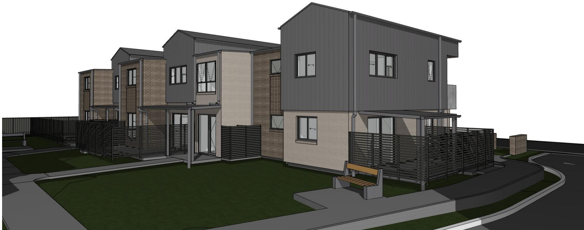
INTERNAL VIEW UNITS 13-18
